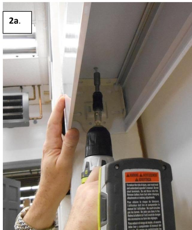
**Step 3: Mount Back Side Channels (follow steps for right and left back side channels)**
