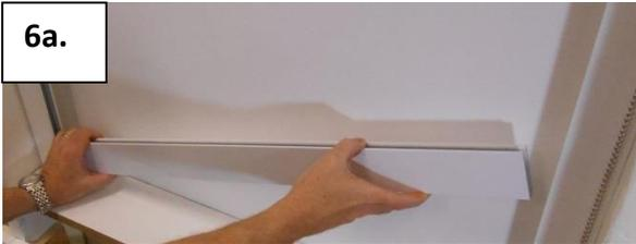
For easier installation, slide light blocking brush up and out of the way while installing the bottom channel.
