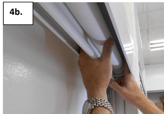
**Step 5: Install Front Side Channel**
