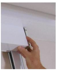
Tip: if you do not have enough clearance to clip the fascia on the top of the bracket, you can slide the fascia over the brackets (if there is enough wall space on the side of the fascia brackets).
