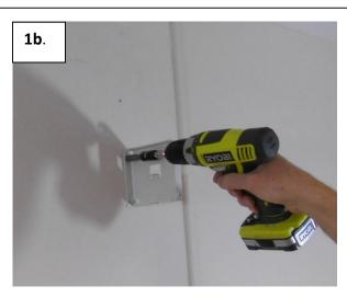
Step 2: Mount Back Side Channels (follow steps for right and left back side channels)
