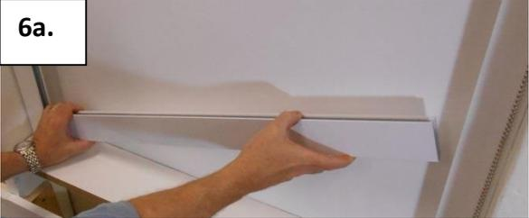
6a. For easier installation, slide light blocking brush up and out of the way while installing the bottom channel.
